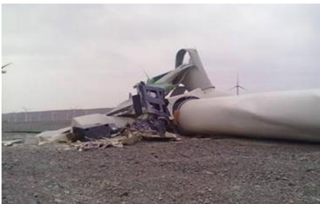
Collapse of an onshore wind turbine unit, on an anonymous construction site in Asia, possibly due to faulty foundation-tower joints during testing at the commissioning stage.
