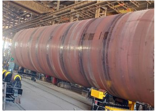
General photographic view, showing a turbine tower, inspected by ETD at the assembly welding stage at an anonymous factory.
