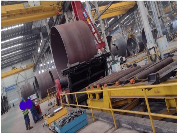
General photographic view, showing a tubular section formed, inspected by ETD at the plate rolling stage at an anonymous factory.
