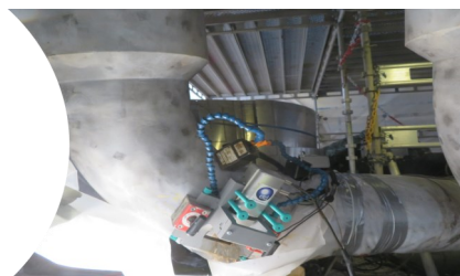
EDSE being used on a pipe elbow
